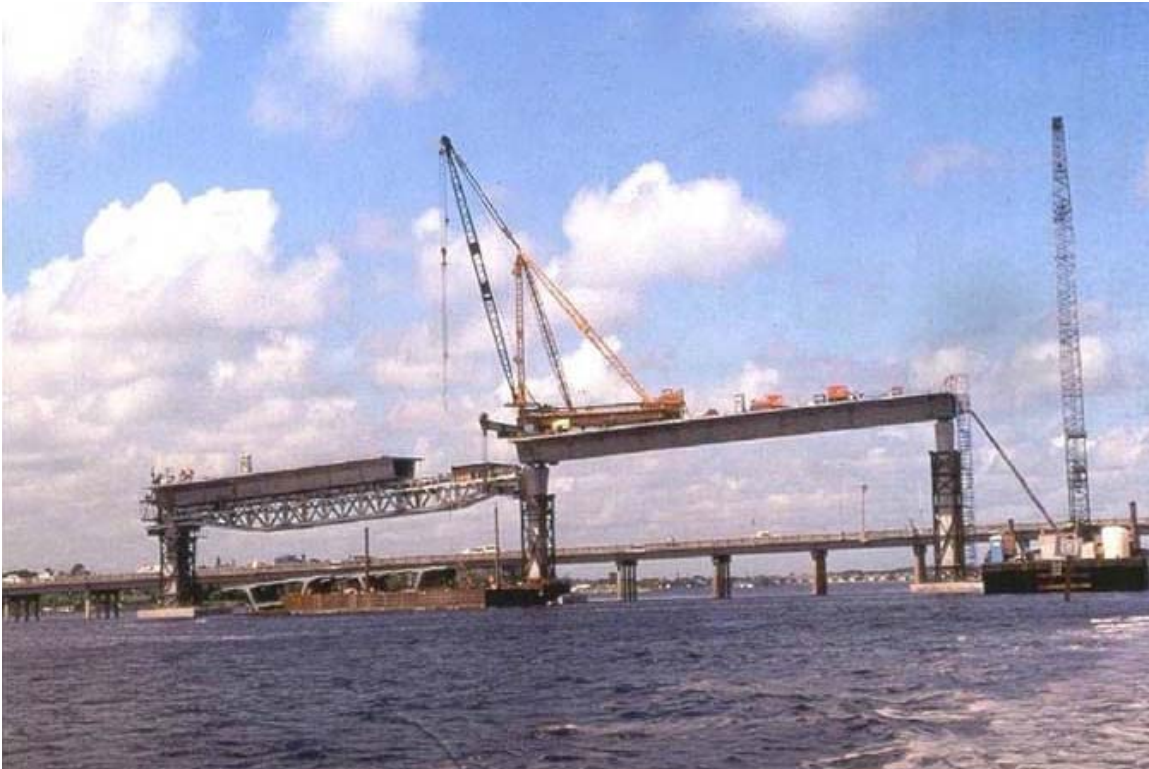
Figure 20.9.2-1 Span by Span Construction
