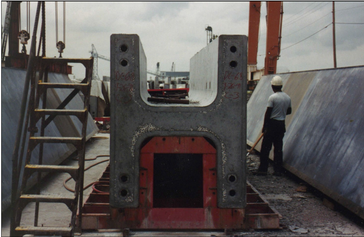
Figure 25.4.3.2-3 C.I.P. Foundation and Precast H-Section Pier Column
