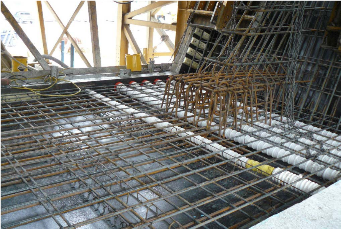
Figure 20.4-1 Reinforcing in Deviation Segment
