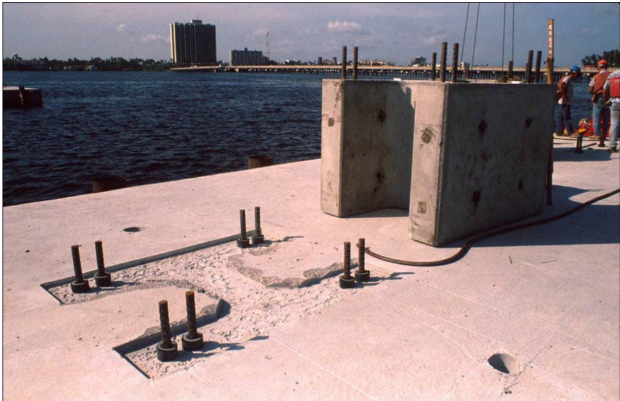
Figure 25.4.3.2-3 C.I.P. Foundation and Precast H-Section Pier Column
