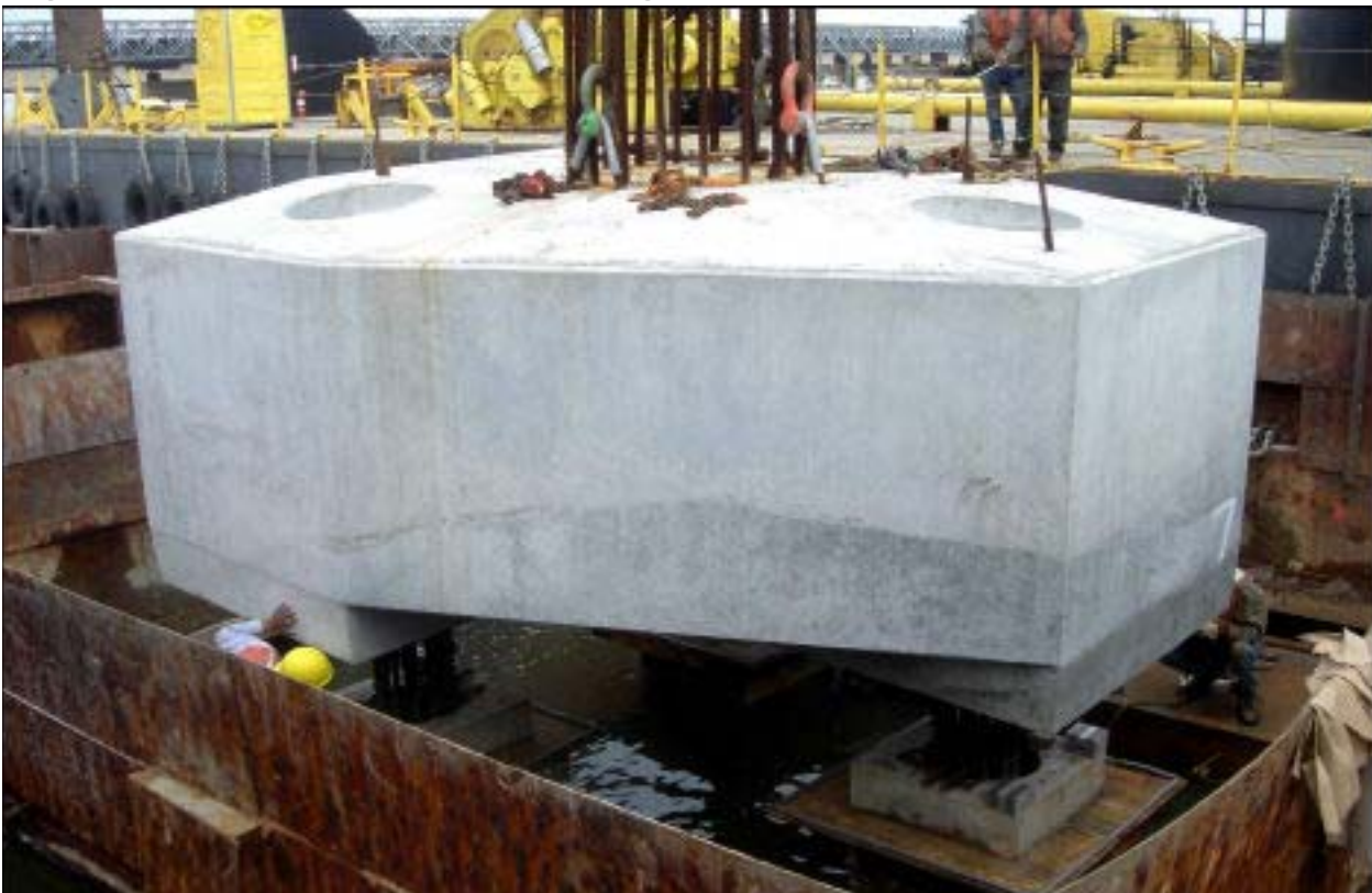
Figure 25.4.3.6-3 Precast Footing Installation
