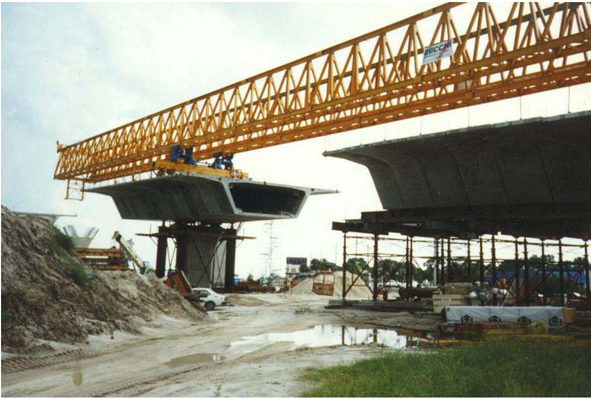
Figure 20.9.1-4 Gantry and Stabilization Towers
