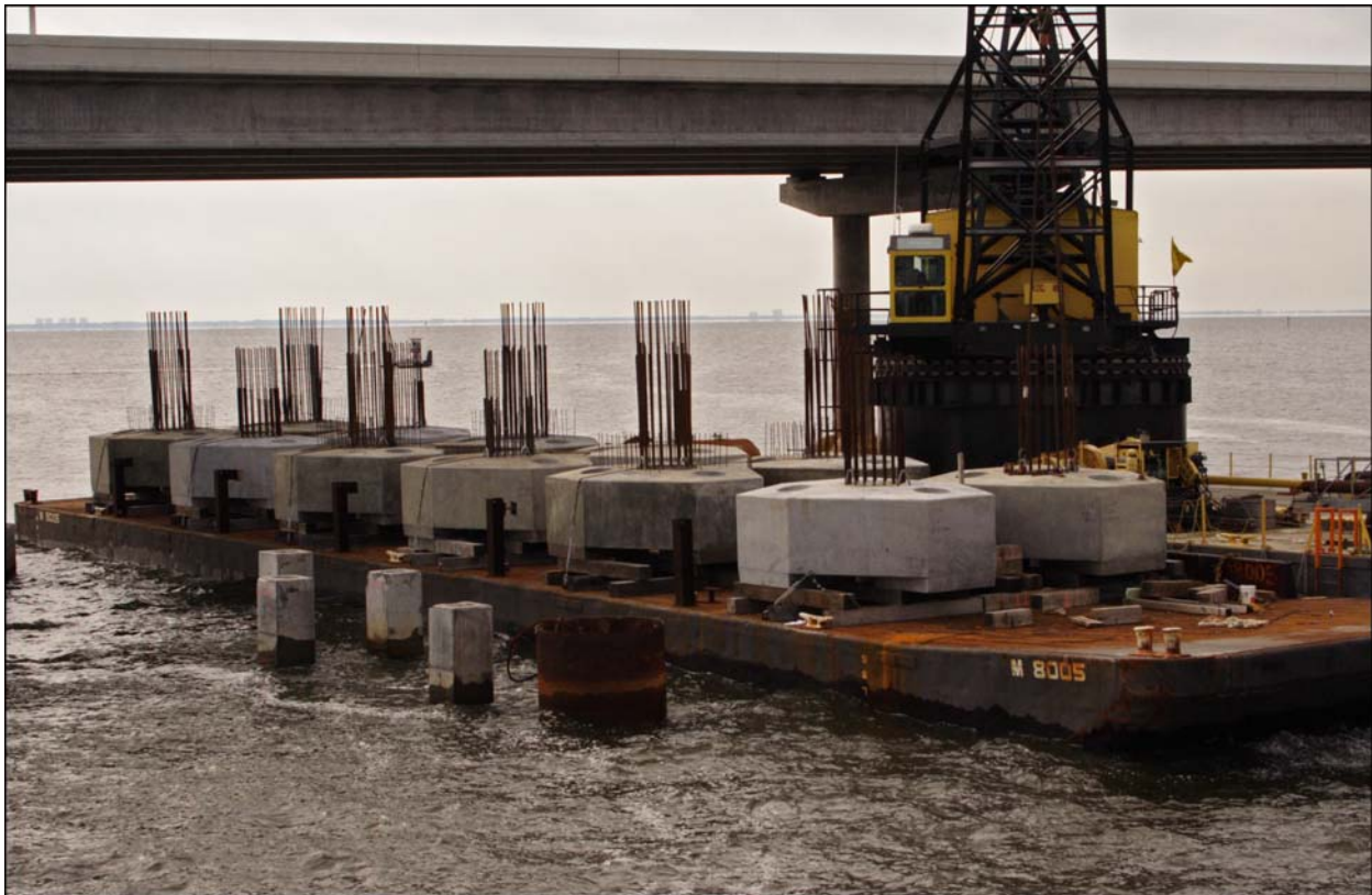
Figure 25.4.3.6-3 Precast Footing Installation
