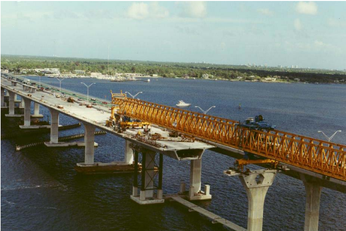
Figure 20.9.1-5 Gantry with Leg on Pier Segment
