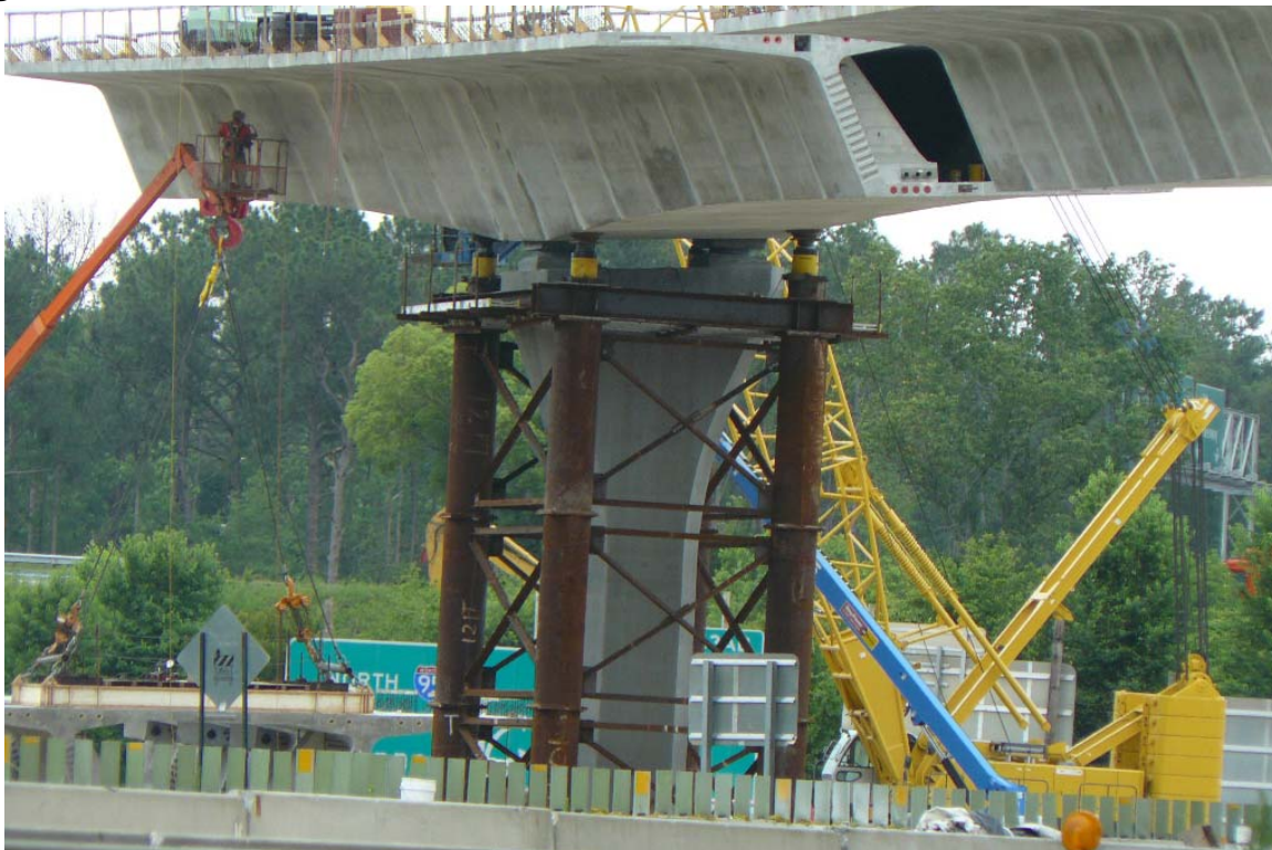
Figure 20.9.1-2 Stabilization of Balanced Cantilever
