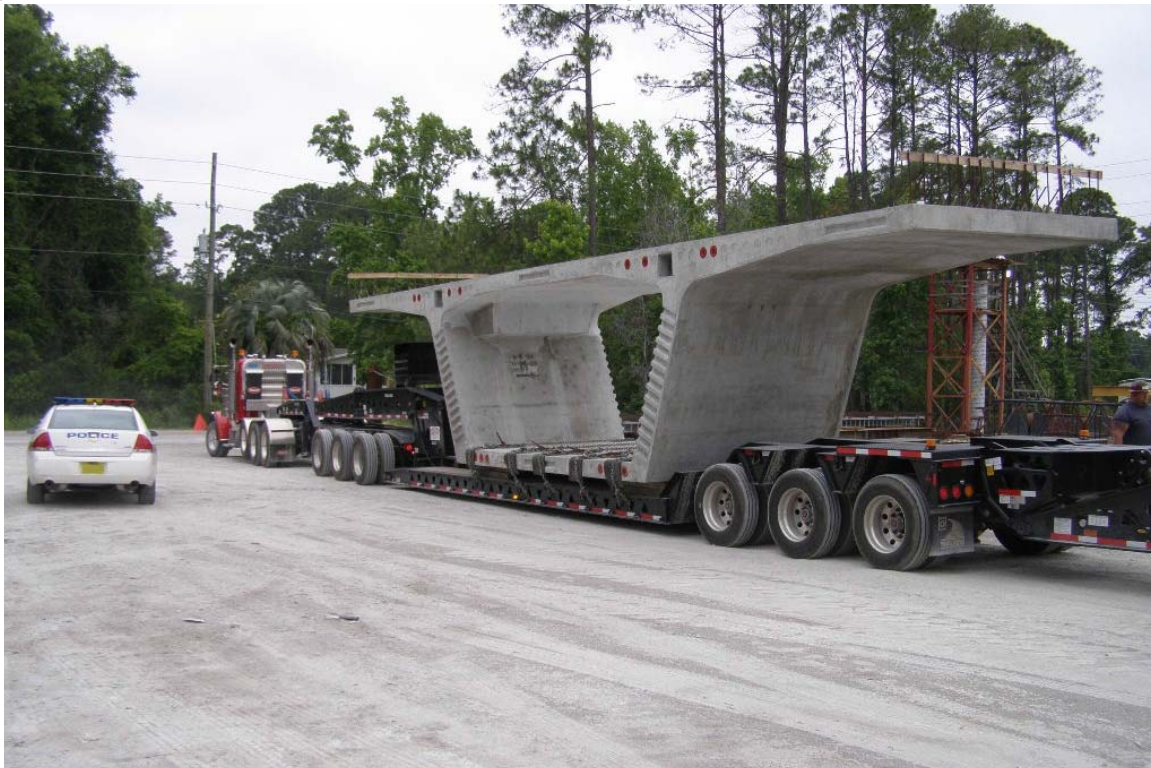
Figure 20.9.2-5 Truck Loaded with Segment
