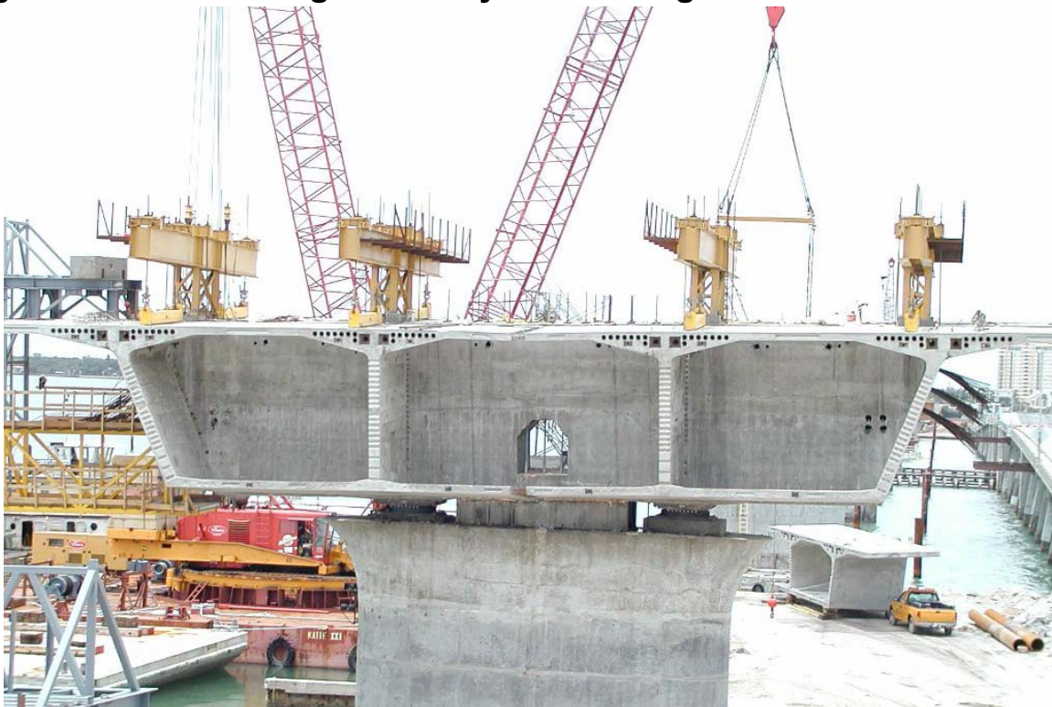
Figure 20.9.1-3 Setting Geometry with Strongbacks
