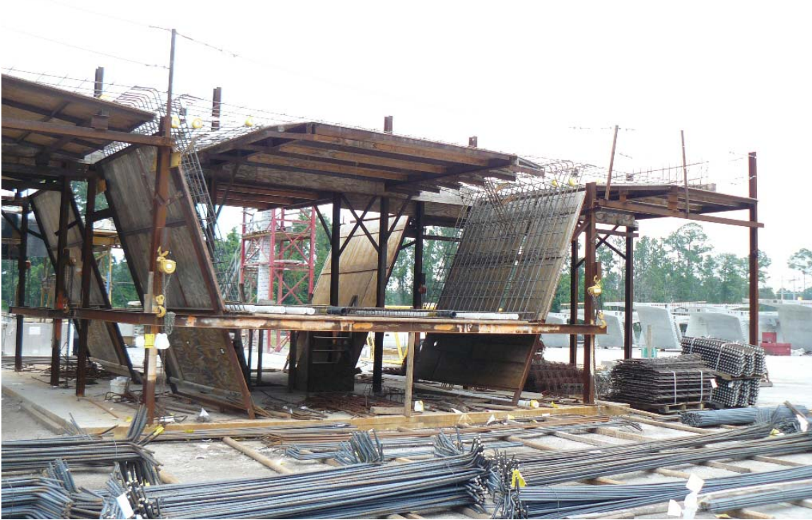
Figure 20.1-1 Reinforcing Jig for Variable Depth Segment
