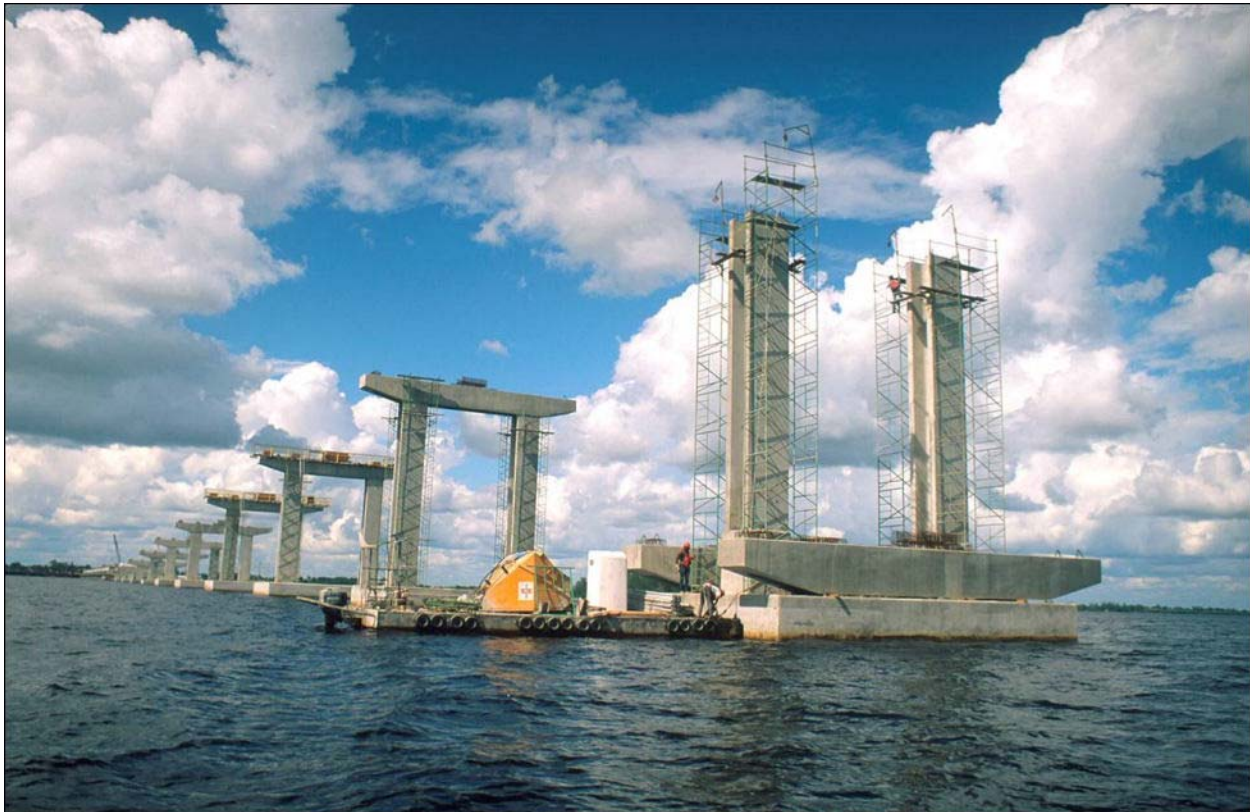
Figure 25.4.3.3-1 Precast Pier Cap Installation
