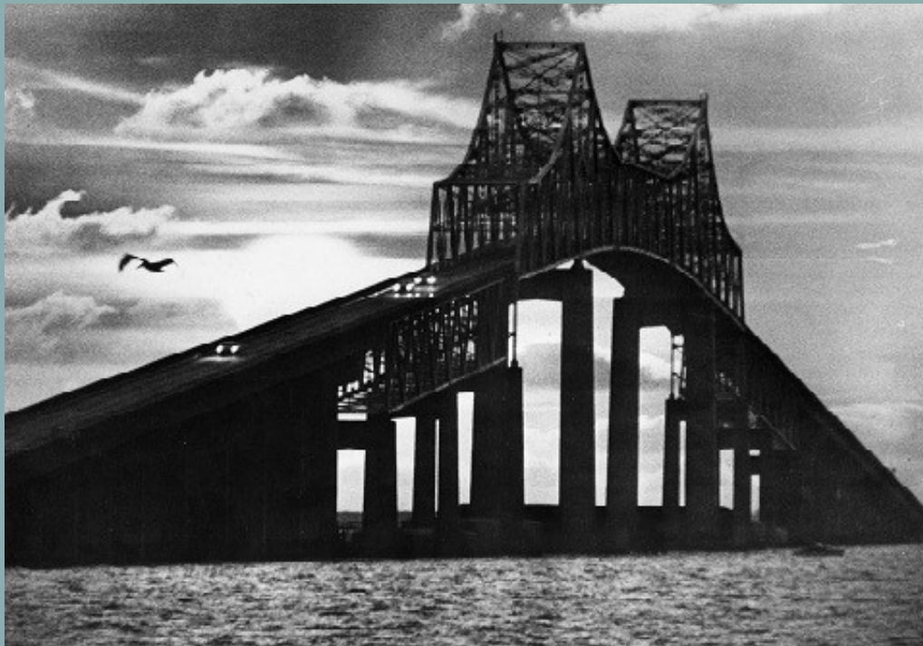
The Sunshine Skyway Bridge connects St. Petersburg in Pinellas County and Terra Ceia in Manatee County, Florida, passing through Hillsborough County waters. (1963)
