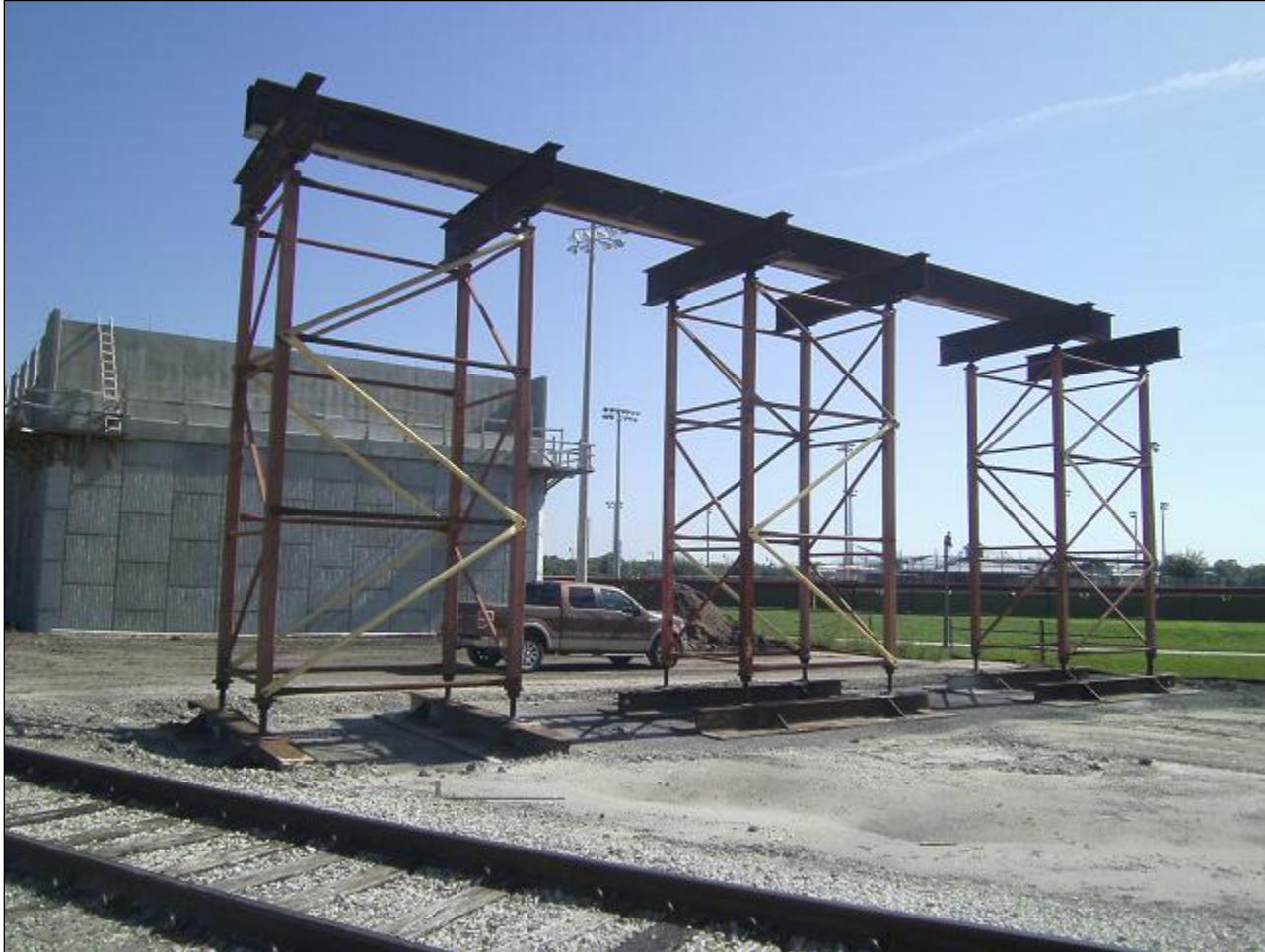
Typical Shoring for a Steel Girder Bridge
