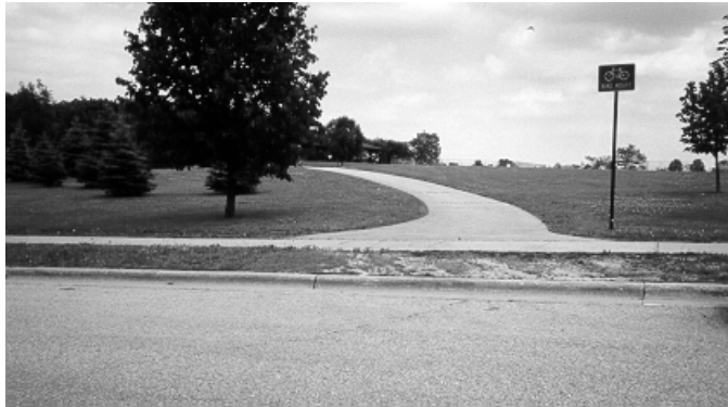
Don't do this. Provide a full width curb cut.
